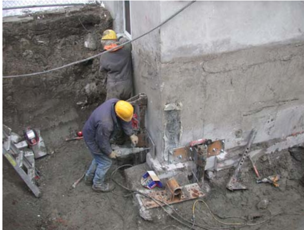
Installation of micro-piles to support damaged foundation in poor soil conditions
