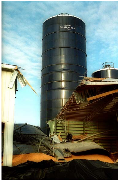
Collapse of a farm silo following a fire
